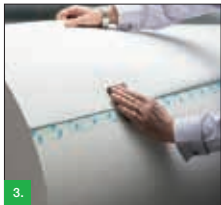
Figure 3: Attach the paper top layer onto the exposed adhesive part of the tape.
