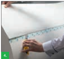
Figure 4: Fold back and remove excess paper tail.
